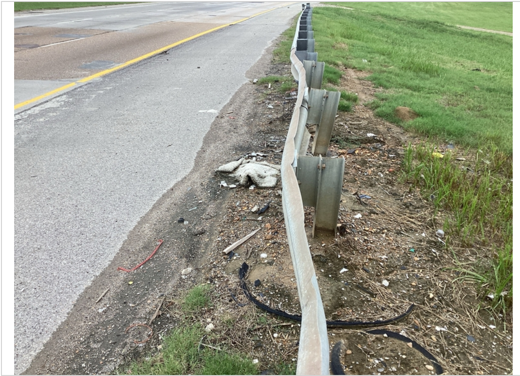
Approach 2 right guardrail damage
