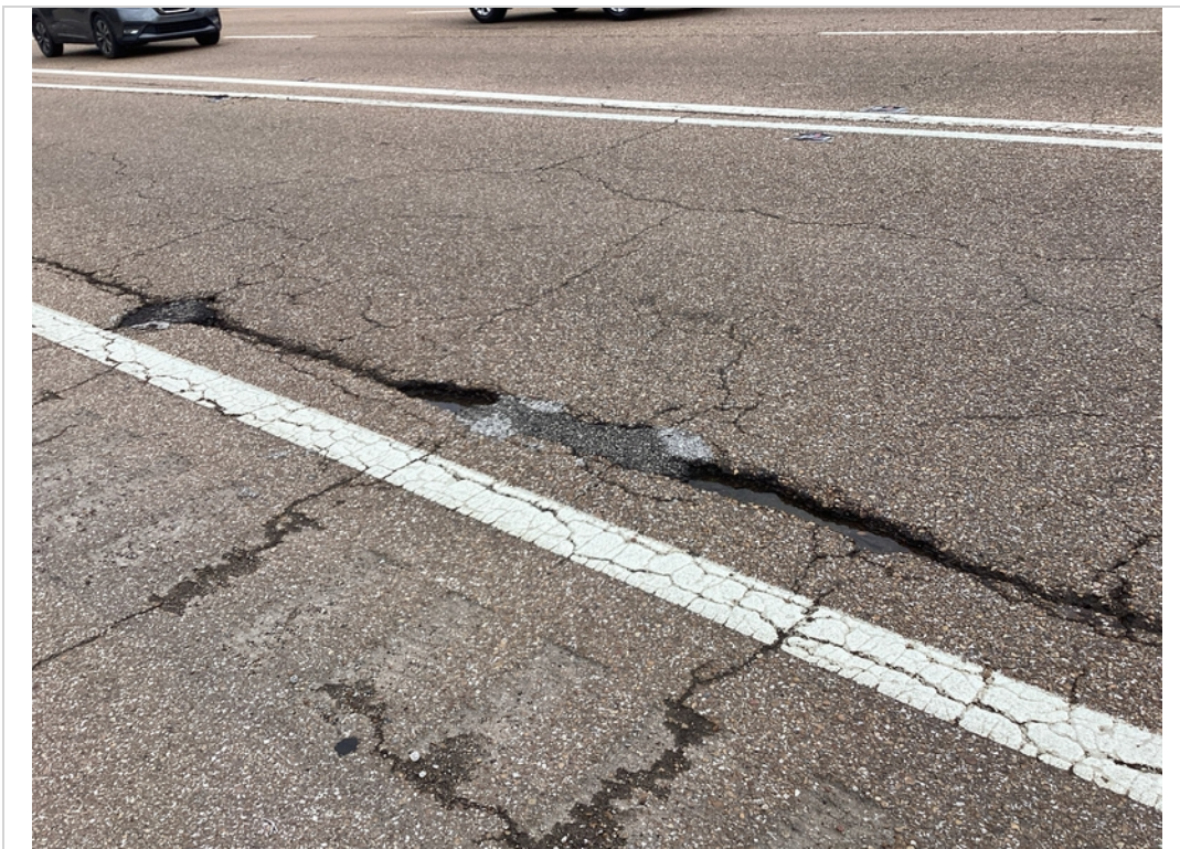
Span 7 top deck spalling/pothole
