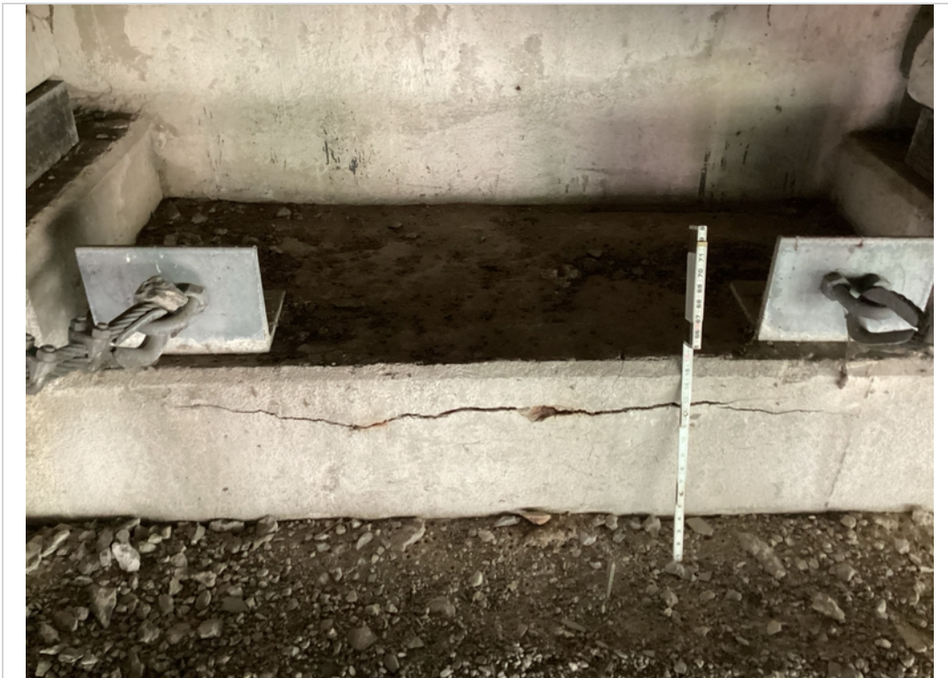
Abutment 1 impending spill
