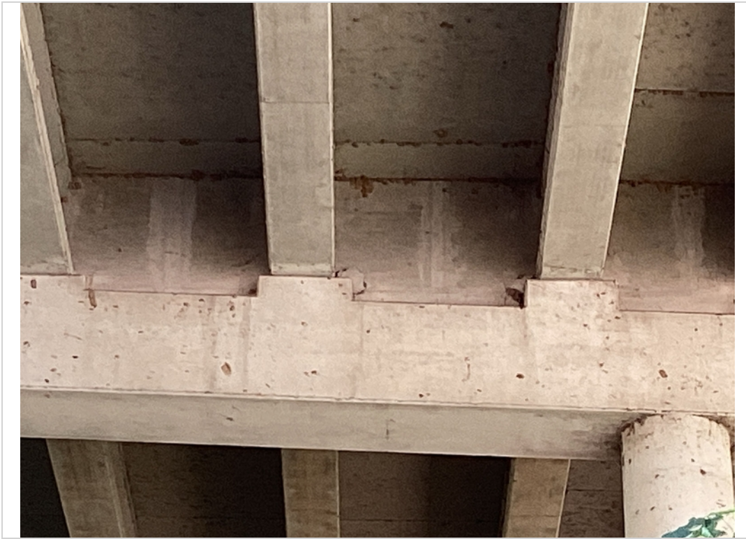
Span 7 diaphragm spall
