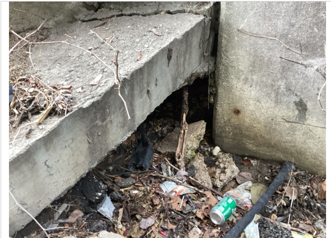
Approach 1 right embankment washing
