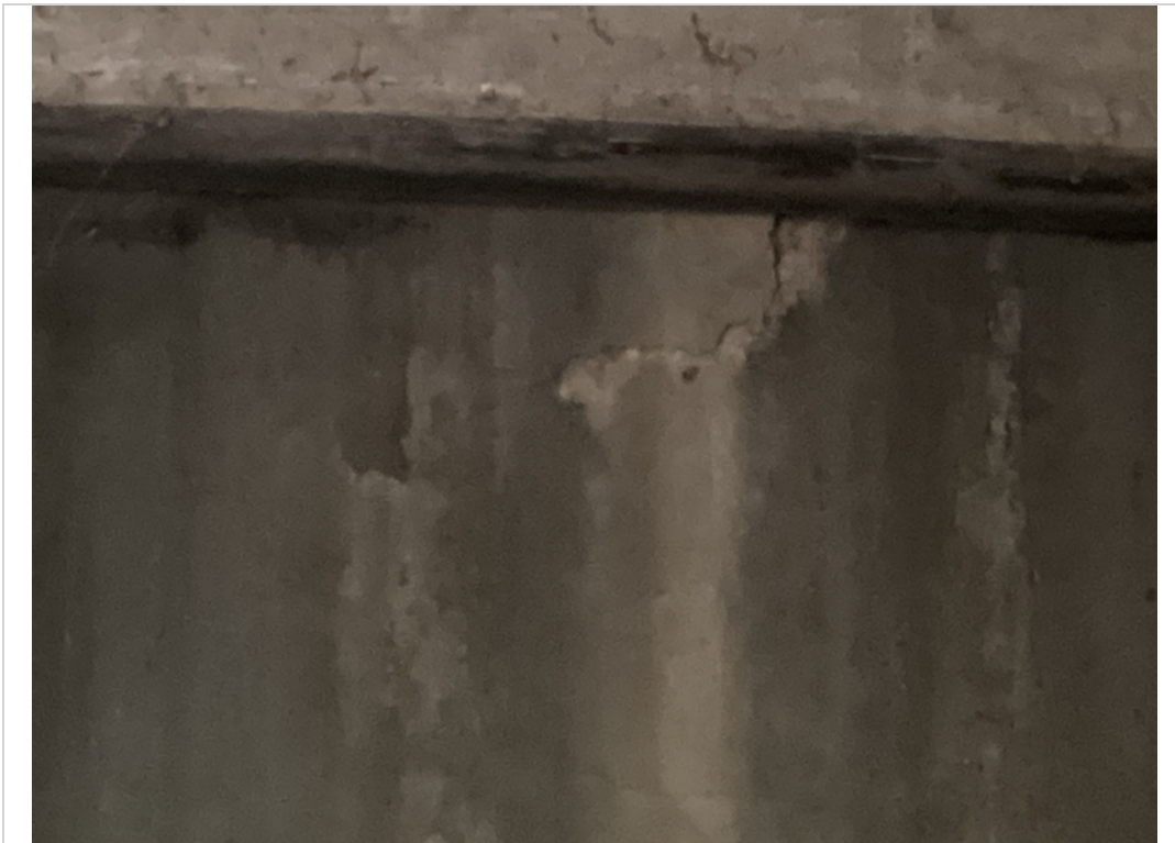
Abutment 2 backwall spall
