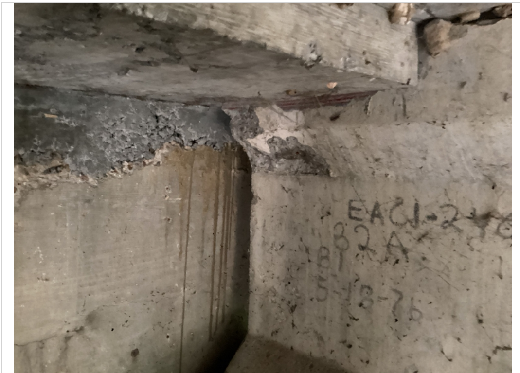
Span 1, beam I, spalling
