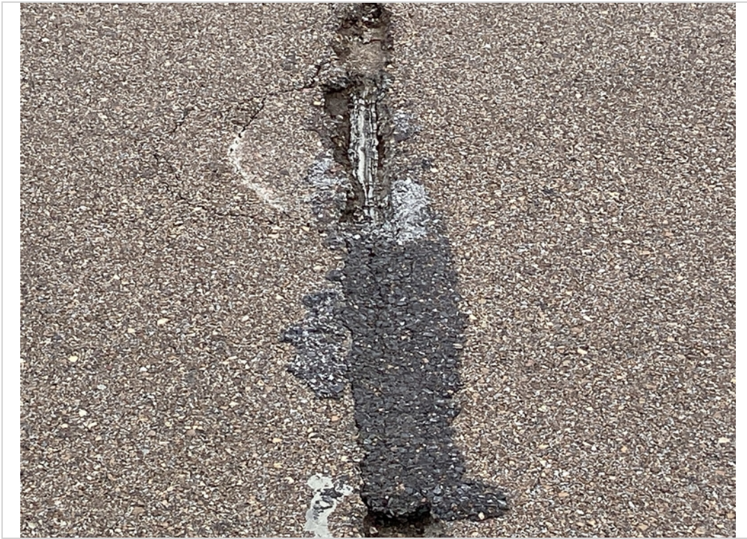
Approach 1 asphalt spill
