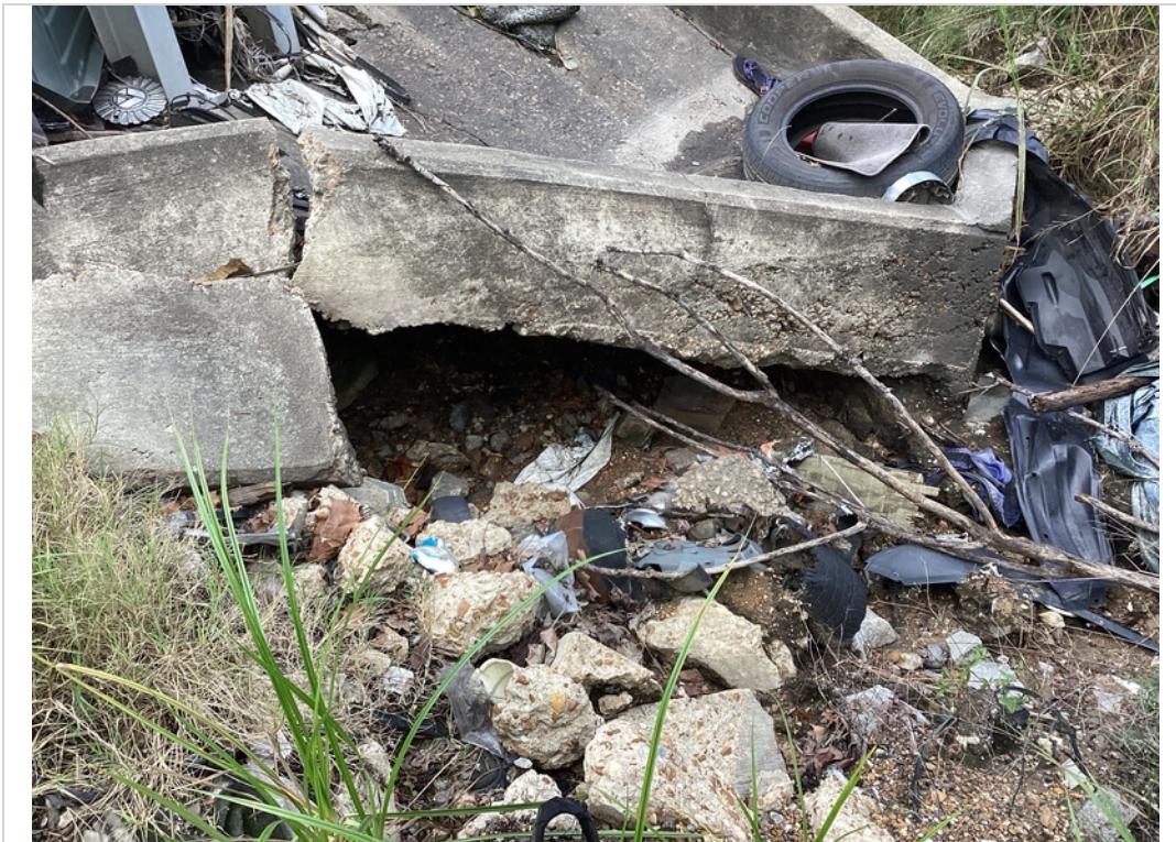
Approach 2 right embankment washing
