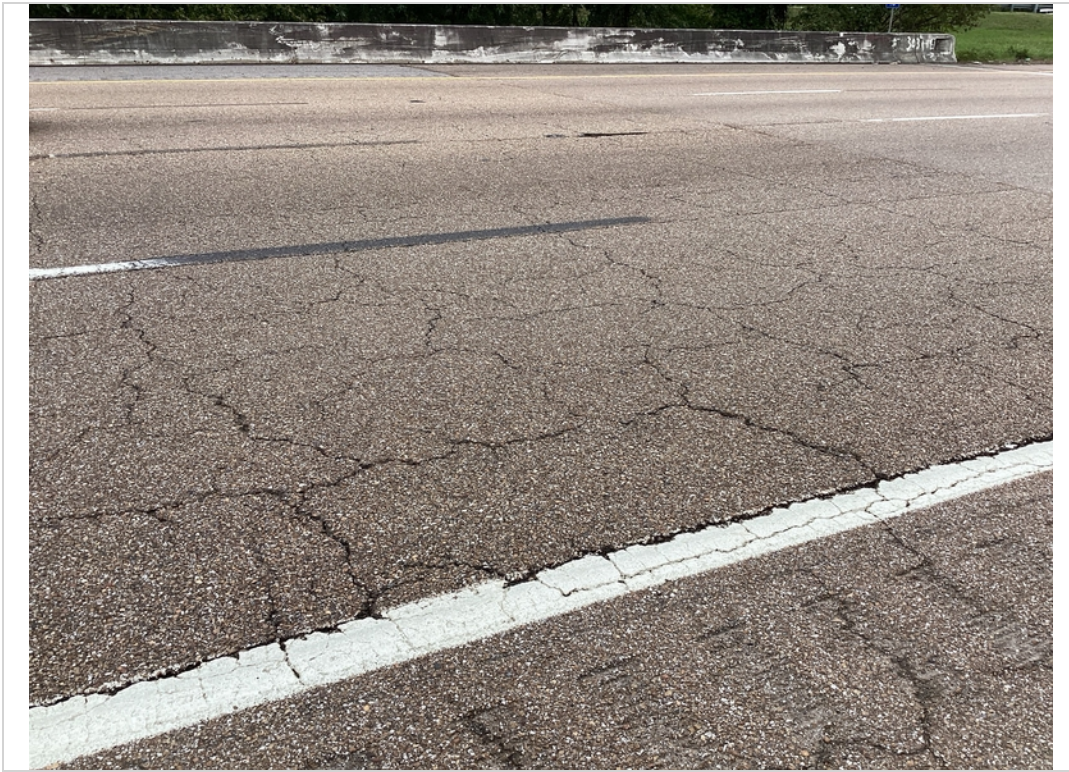
Span 1 cracks & pot holes
