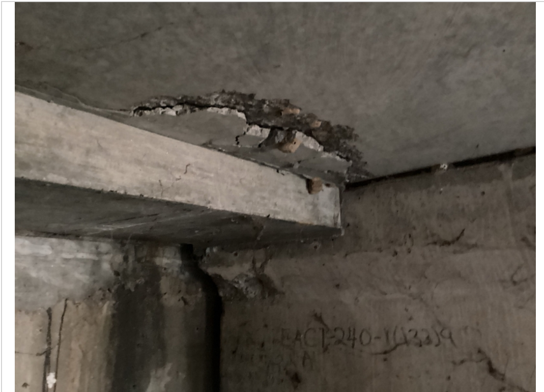
Span 1 , beam H, spall to steel ,bottom deck , impending spall
