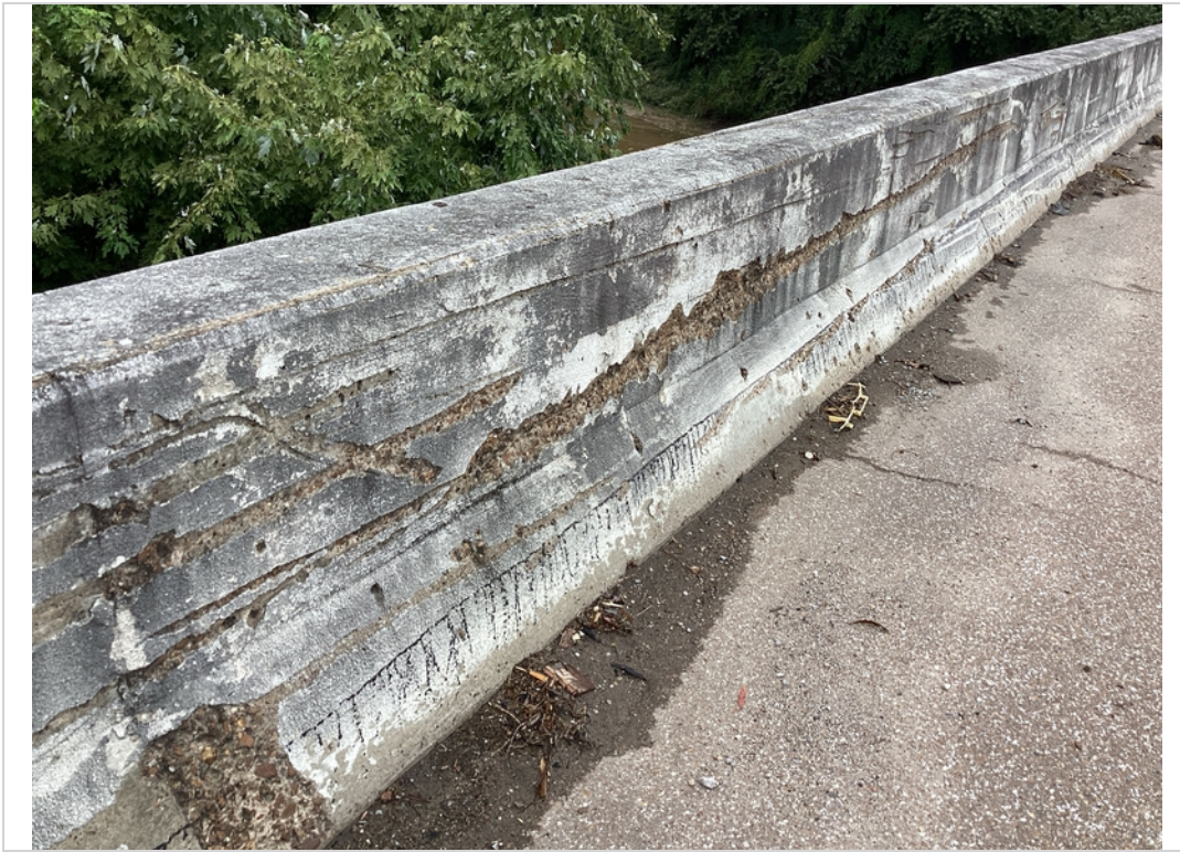
Span 3 parapet , collision damage
